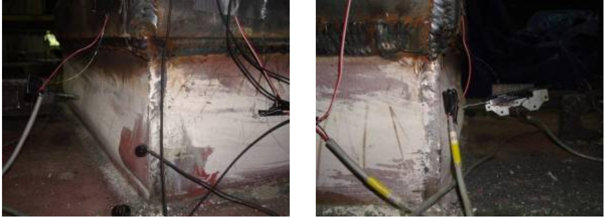
Figure 8. Local Buckling of West Column (West Side) at 1.8% Drift
