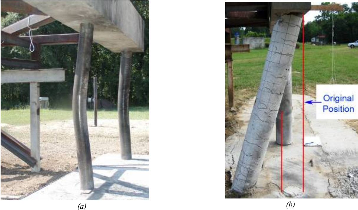
Figure 12. (a) CFST column (D = 127 mm) after the test; (b) RC column after the test
