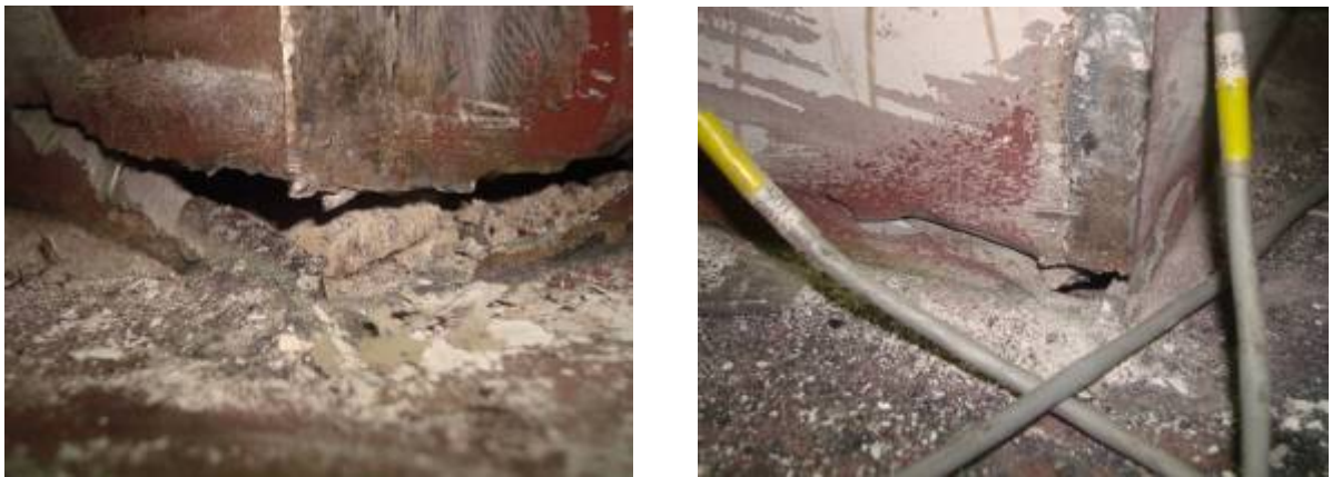
Figure 9. Fracture of West Column (North West Corner) at 2.3% Drift
